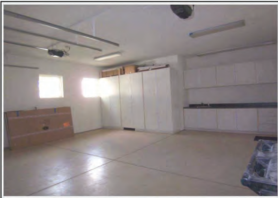
One of the two finished garages with built-in storage and sink
